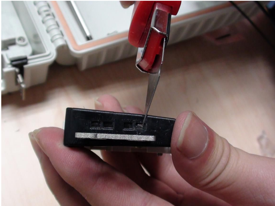
Cut the rubber as the way in the picture. *This example is for the preconnectorized drop cable
